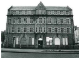
The old lodging house, renovated to become Langstane's Peacocks Court, Aberdeen
